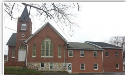
The addition Minghini's constructed is shown on the right in this photo.
