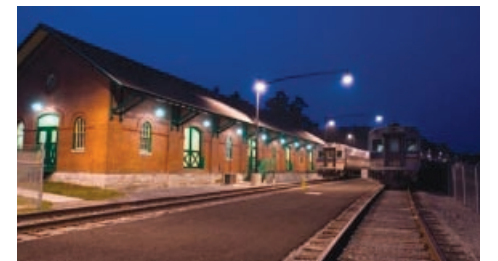
2005 ABC-CVC Award of Excellence Winner: the CSX MARC Layover facility built by Minghini's.
